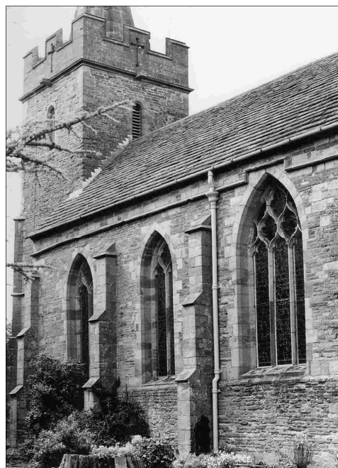
Fig. 2. Dinmore chapel, showing reticulated tracery.
